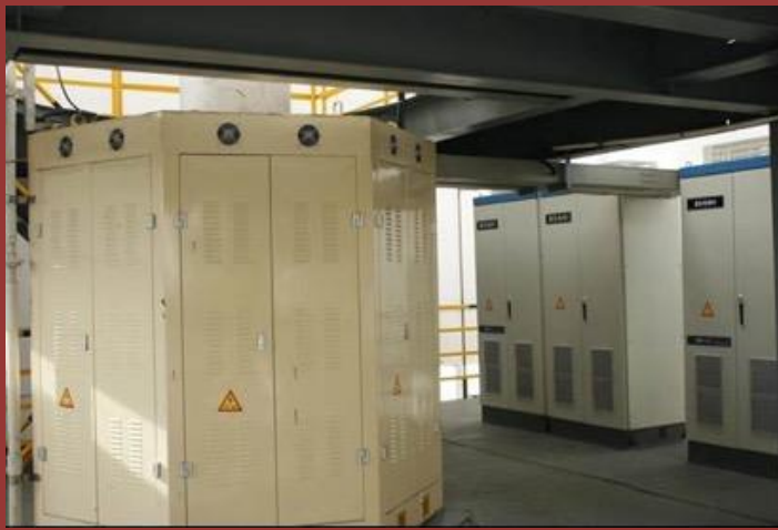
Figure 4: HCl solution purification equipment with microwave energy
