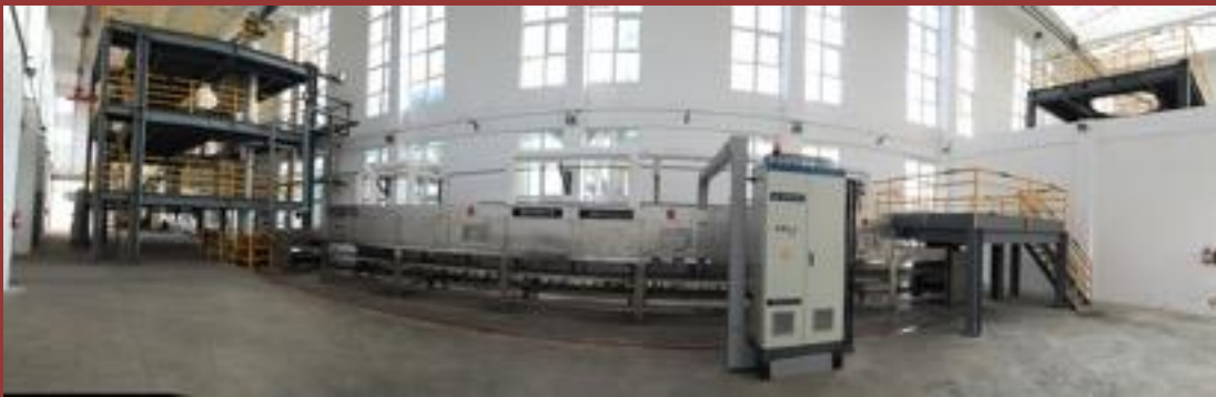
Figure 6: The whole system view of the MW Cl removal process
