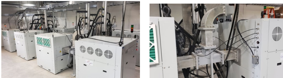
Figure 2. (a) View of the eight Crescend Technologies PrecisePower™ PTL-50 solid state microwave generators. The vertical risers are part of the water cooling system. (b) The power
